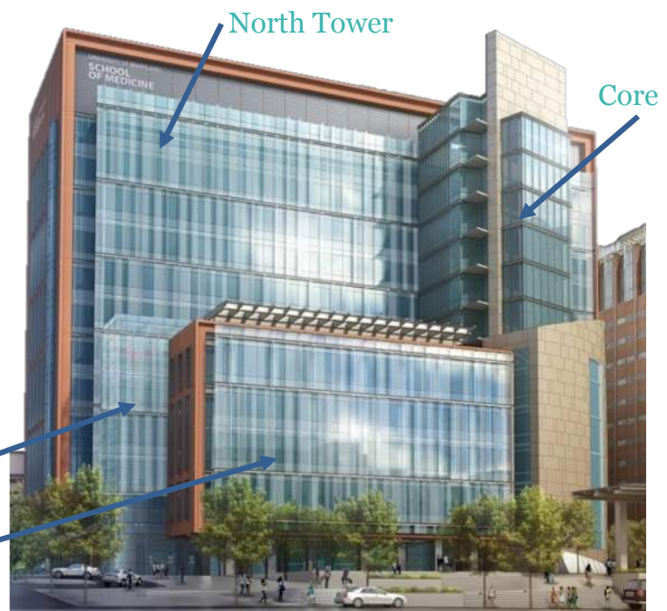
Figure 1: South view of HSFIII
